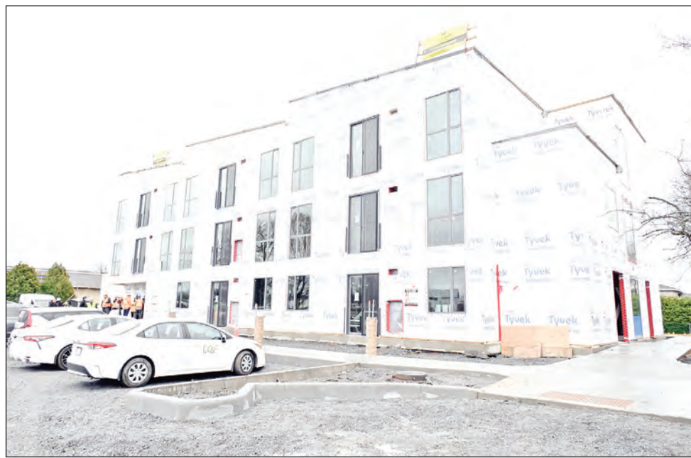
The exterior of Morrisburg's new Morris Glen Court apartment complex leaves no question that it is still under construction, but as cladding and masonry is added in the coming months, the appearance will change quickly. Tinkess Photo
